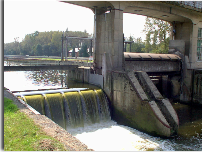
FIGURE 2. Automated control gates in the Sambre river (Belgium). The left gate is in operation. The right gate is lifted for maintenance. (©L.Moens)
